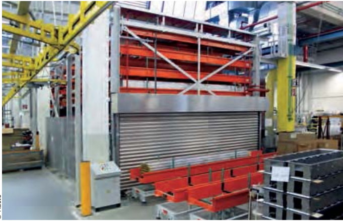
© Kasto The access area of the Unitop storage system in the basement of the factory building of Zumtobel Lighting
